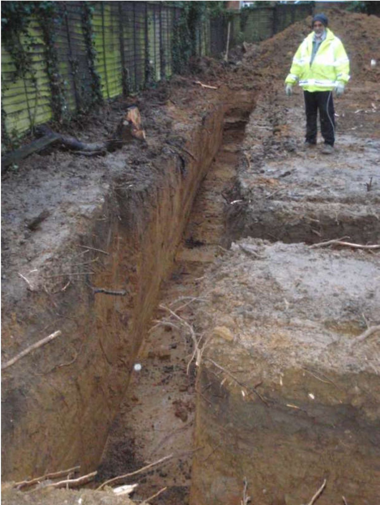
Plate 3. The site showing cutting of foundation trenches on the east side
