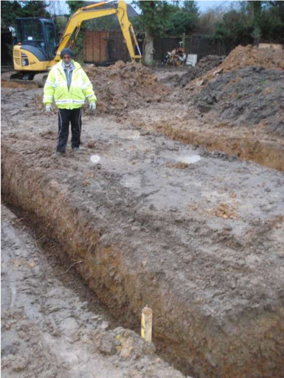
Plate 4. Foundation trenches on the west side
