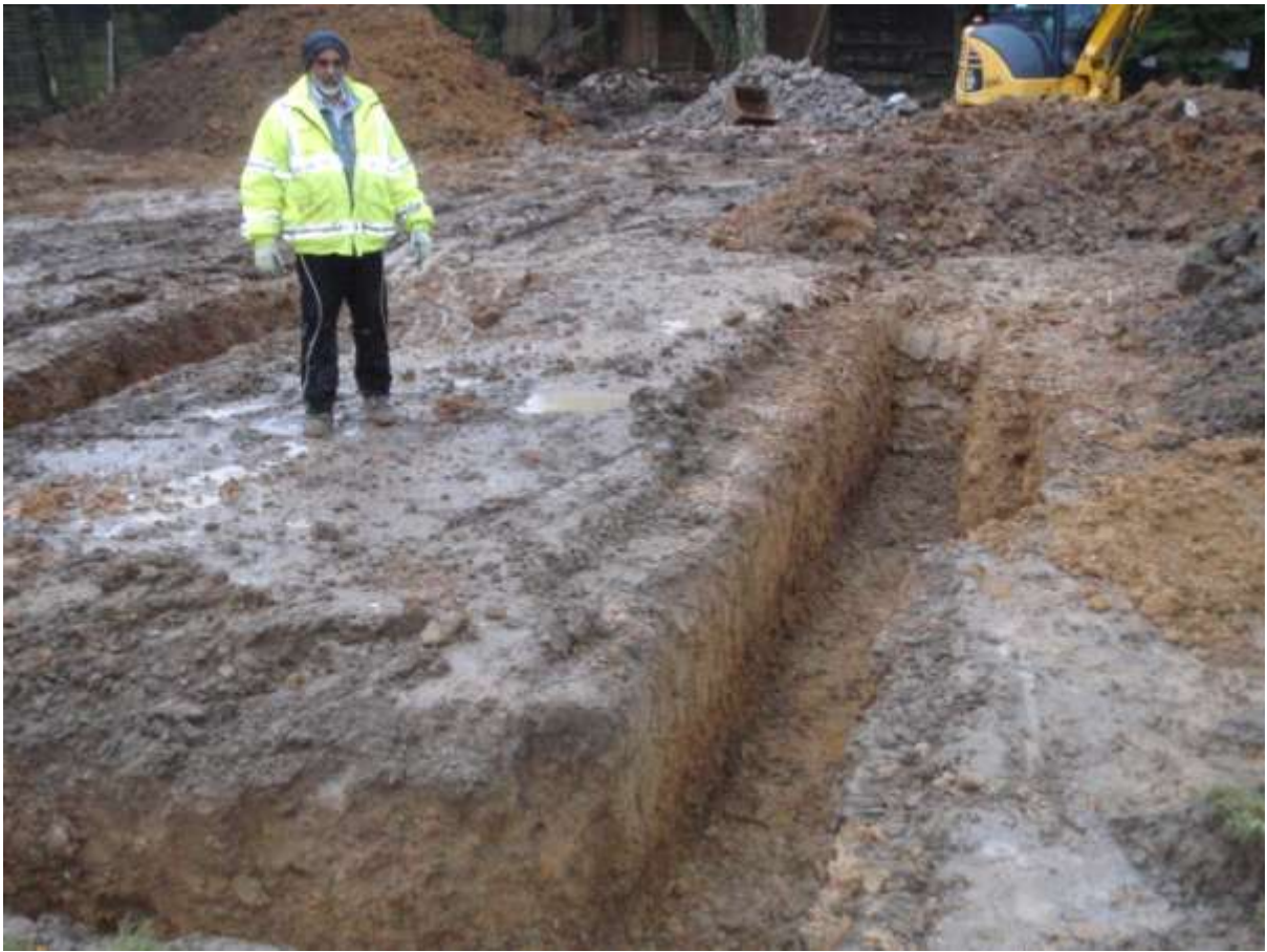
Plate 2. General view of site, facing south-east
